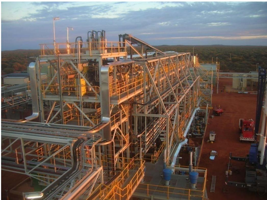
**The Flotation section of the Concentration Plant**
